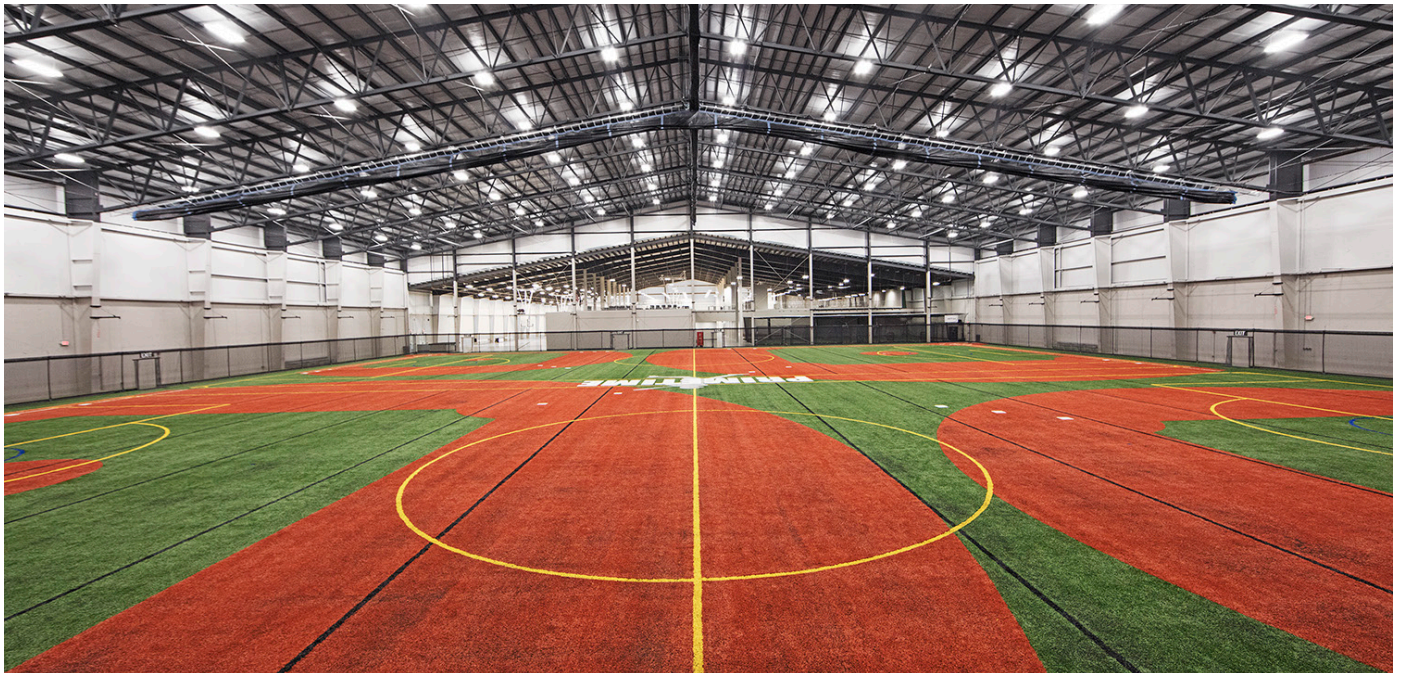
The exterior metal panels and roofing are prefinished, including a 245-foot span over the turf area with no interior columns for support.
